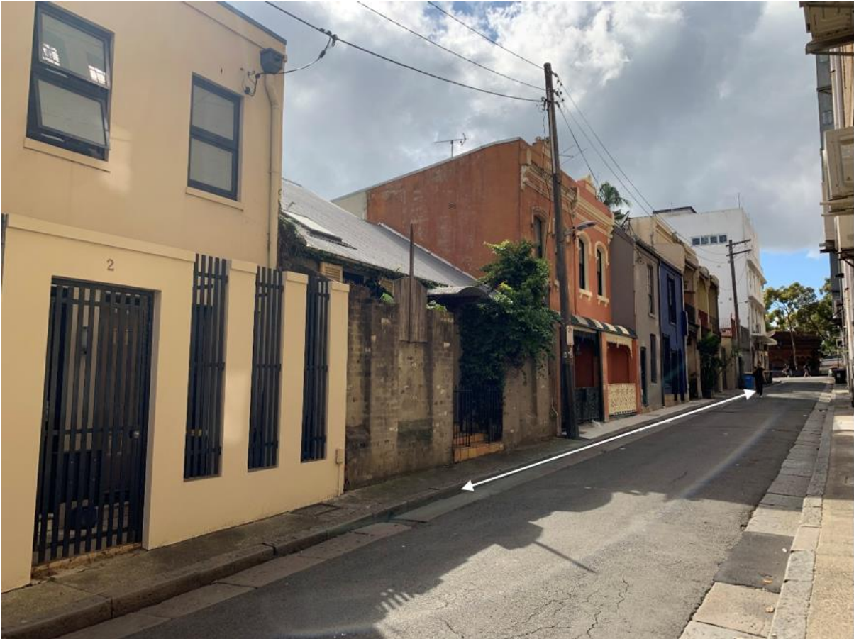
Figure 4: Development to the north at 4 to 18 Foley Street
