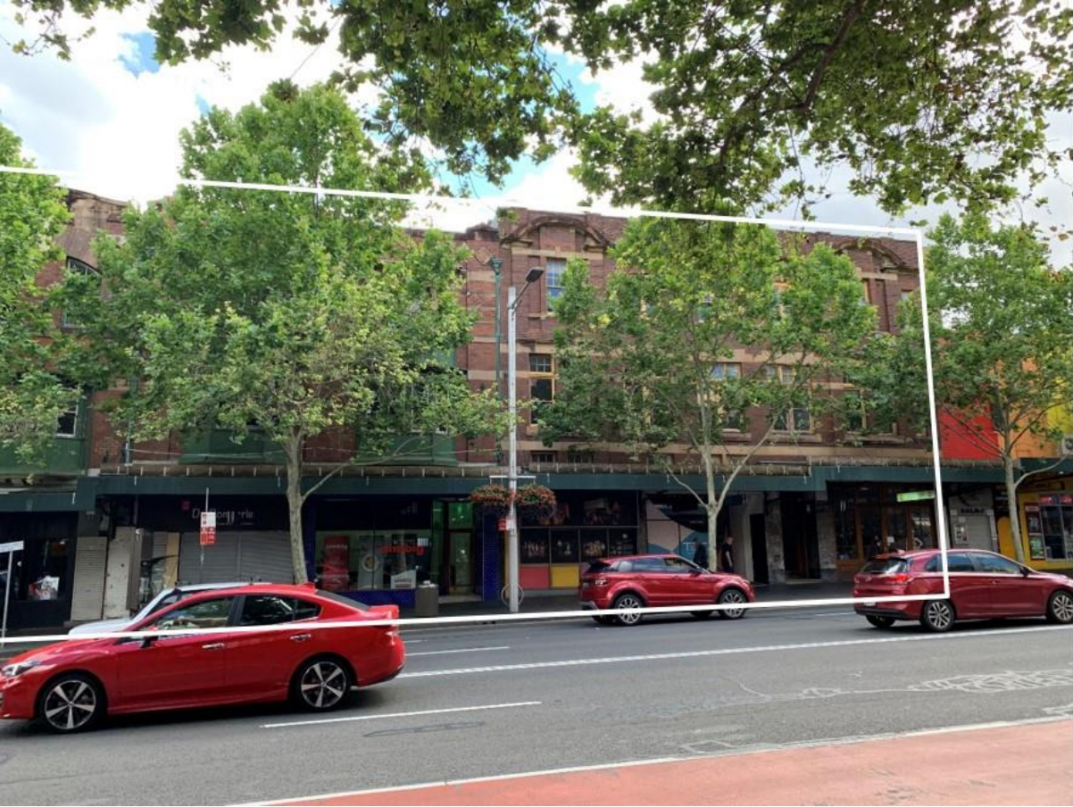
Figure 2: Site viewed from Oxford Street (prior to the installation of hoardings)
