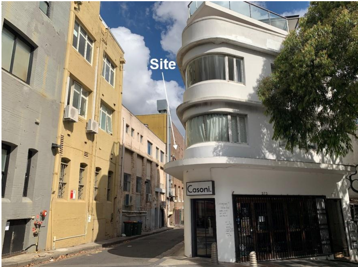
Figure 5: Foley Street as viewed from Taylor Square
